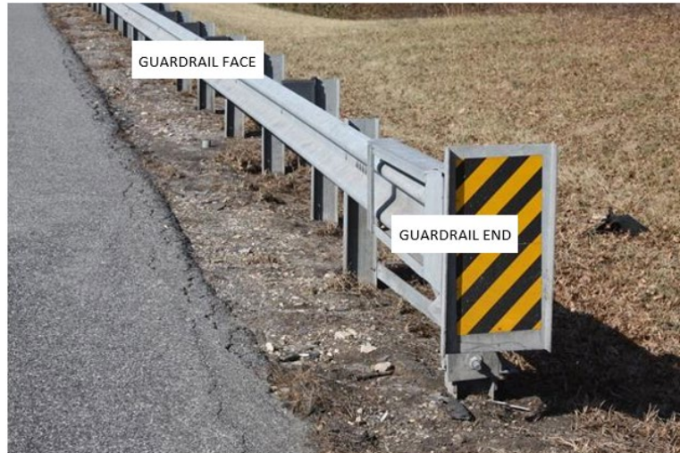
Figure 1. Guardrail face and guardrail end. Source: FHWA
