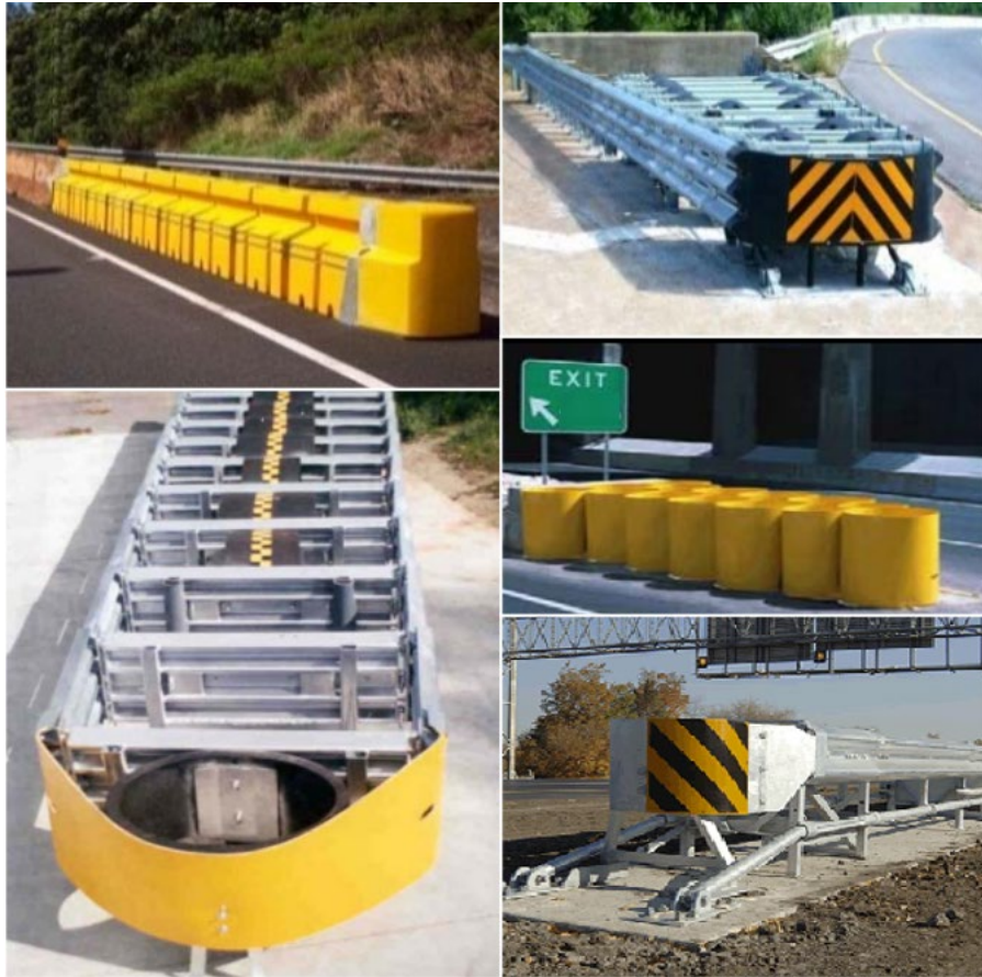
Figure 2. Impact attenuator or crash cushion. Source: FHWA
